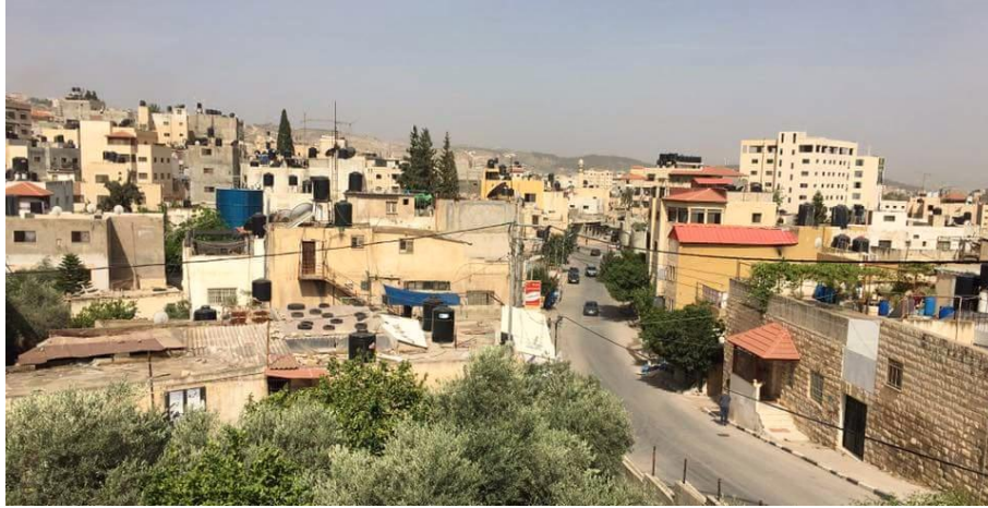
Picture 7-5: Neighbourhood with unacceptable quality of the buildings physical conditions - quarter 17
