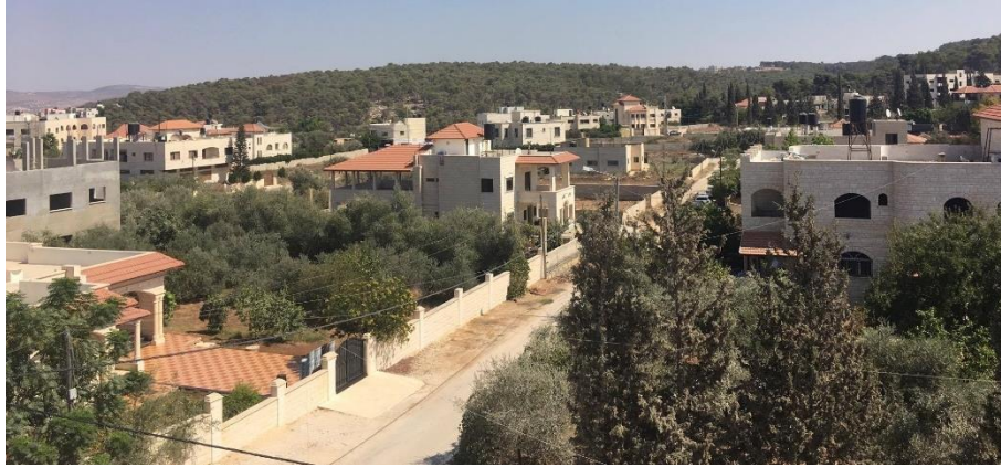
Picture 7-7: Neighbourhood with very acceptable quality of the buildings' layout - quarter 28
