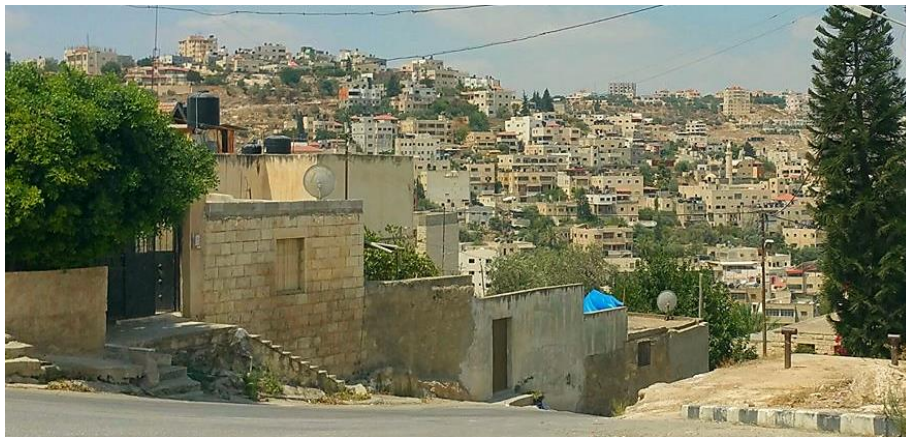
Picture 7-4: Neighbourhood with moderate quality of the buildings' physical conditions - quarter 26
