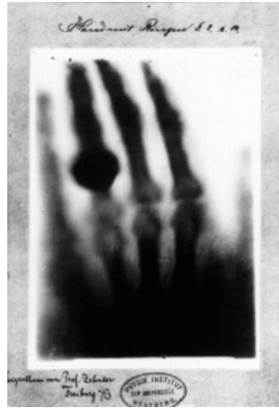
Figure 2.1.: The first x-ray projection was taken in 1895 from Prof. Wilhelm Röntgen's wife which was recorded on a film, showing the finger bones and her ring [Kev98].
