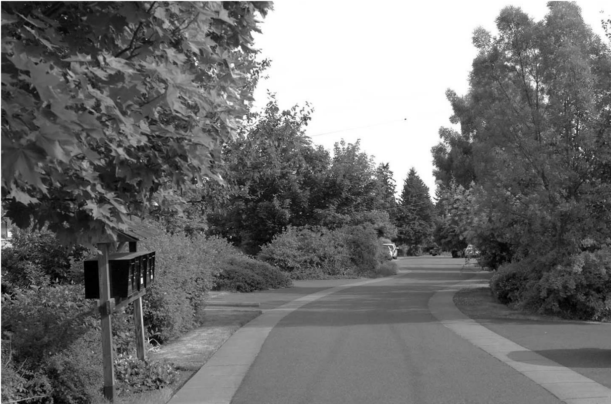
Fig. 5: The “Street Edge Alternative” in Seattle is often referred to as an early example of green infrastructure targeted at storm water management. Roads in residential areas have been redesigned to retain stormwater, but with co-benefits such reduced traffic speed and increased aesthetic quality through reducing road widths and planting (own photo from 2013).
