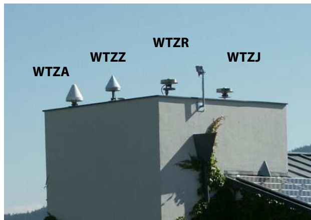
Fig. 5.1: GNSS permanent sites on top of the tower of the main building of the Geodetic Observatory Wettzell. A webcam to monitor snow coverage of the antennas is mounted between WTZR and WTZJ.
