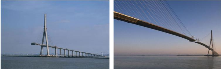
**Figure 4.12:** *Pont de Normandie* (France), during construction in the cantilevering phase and before juncture of the two free ends
