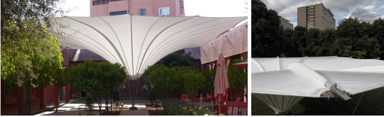
**Figure 4.5:** *Umbrella for Marrakech*: Finalized structure and detail of inclusion of the bent arms (©J. Lienhard [85], used with kind permission)
