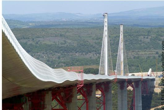
**Figure 4.13:** *Viaduc de Millau* (France), showing considerable deformations in the bridge deck during incremental launching (©CEVM Eiffage / Foster+Partners / JL DERU – photo-daylight.com, used with kind permission)
