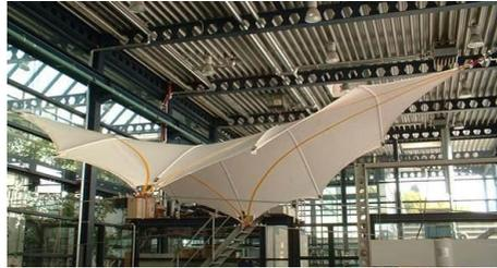
(b) *Bat-sail* developed by Off [107] with integrated GFRP rods to increase the covered area (©Robert Off / IMS-institute, with kind permission)
