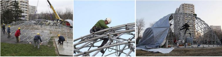
**Figure 4.3:** Ephemeral Cathedral of Cr eteil – a gridshell in FRP constructed through elastic bending: Lifting of the grid, bracing by a third layer and covering with a PVC-coated membrane
