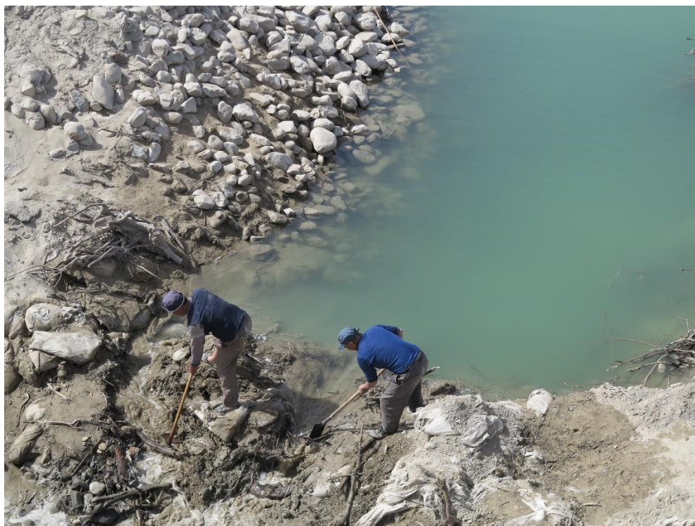
Figure A12: Unauthorized water abstraction. Water surveillance is a difficult issue along the river of 1321 km.
