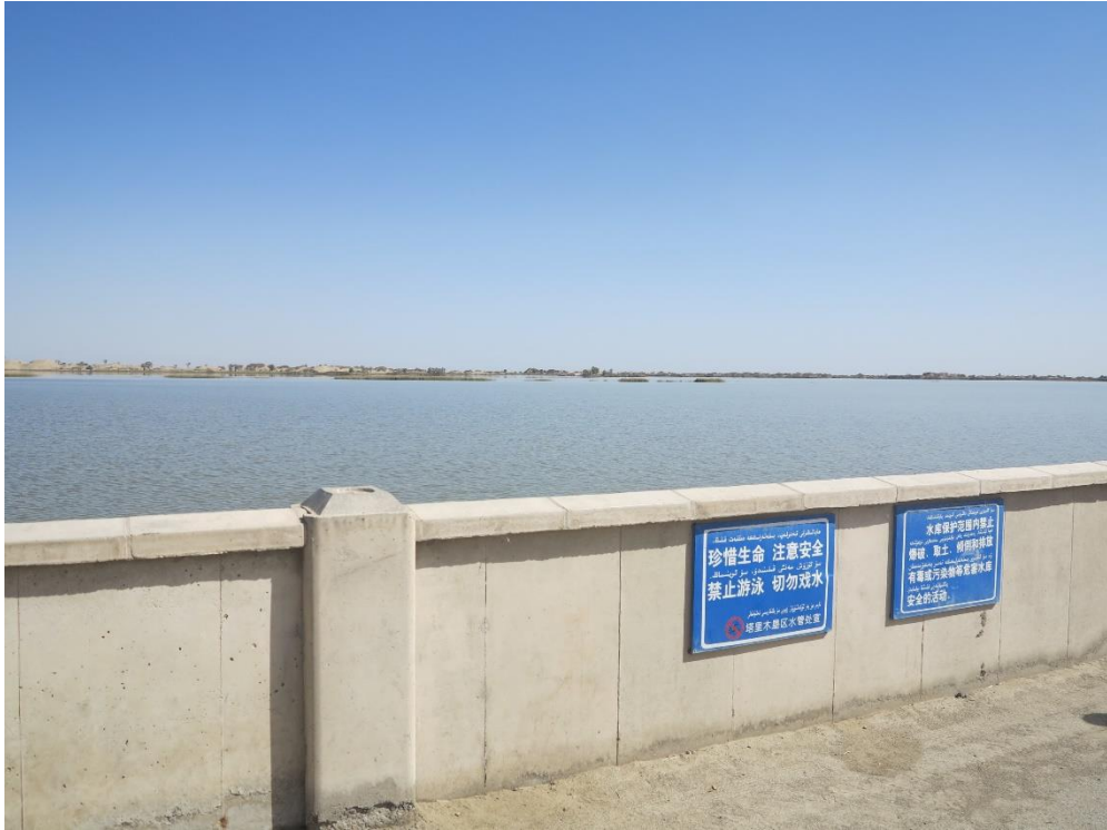
Figure A13: Qiala Reservoir. The largest reservoir in lower reaches.
