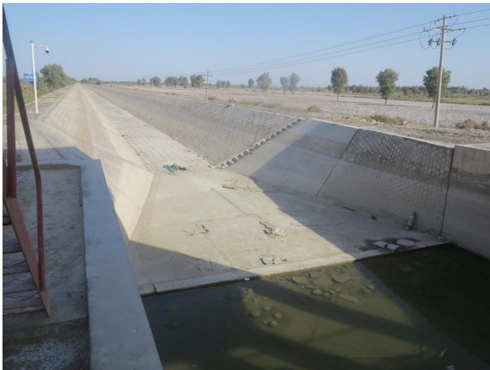
Figure A7: Dry canal in the lower reaches.
