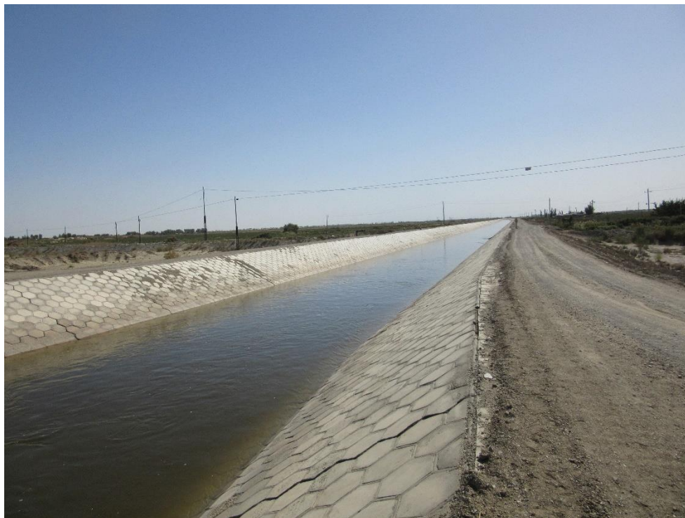
Figure A11: Water-tight canal in lower reaches. New canals and river banks have been built in recent years to prevent water losses.
