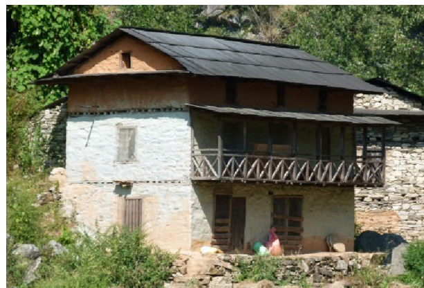
Fig. 9. Hill house in Dolakha with shaded terrace and balcony.
