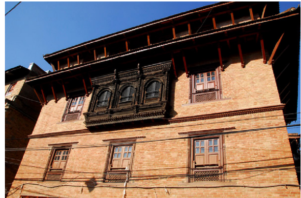
Fig. 10. Façade of Newar house with big wood carved window and large roof overhang.
