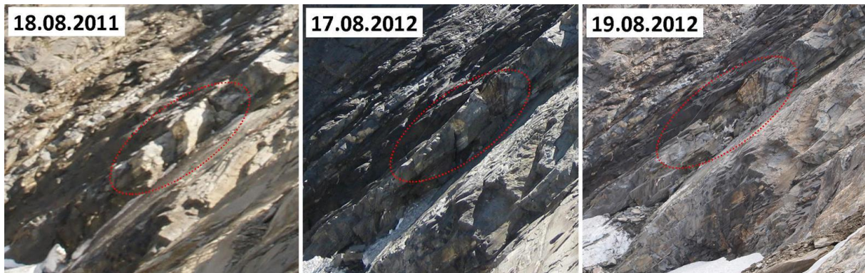
Figure 59: Detachment of the blockslide: 18. August 2011 (left) - intact rock, 17. August 2012 - crack visible in the tensile zone (middle), 19. August 2012 – situation after the release (right).
