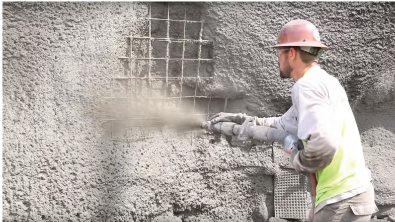
Figure 28: Application of shotcrete, cited from [164].
