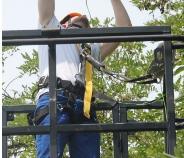
Figure 9: An example of how the safety gear is used correctly.
