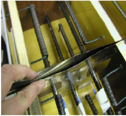
Figure 3-6: Stainless foils are prepositioned in
