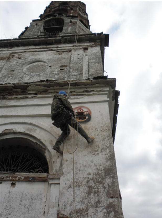
m. Sample C20, two bricks above C14
