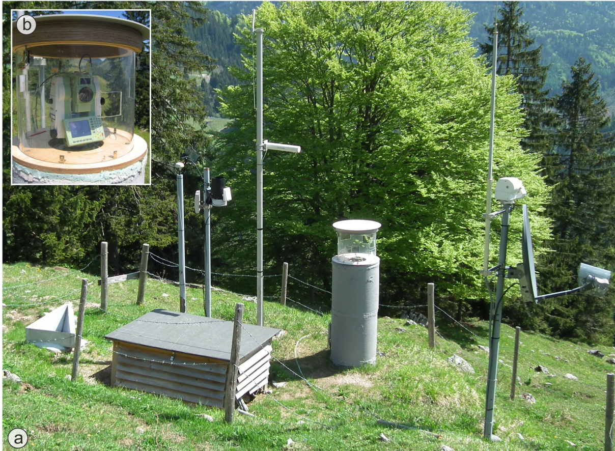
Figure 31: a) Photograph of the alpEWAS main sensor node located on the middle part of the landslide. On the far left pole the GNSS receiver is mounted, on the poles to the right follow the weather station and on the next one the directional antennas ensuring the connection to other GNSS sensor nodes. The VTPS (inset b)) is installed on the pillar and a webcam and a satellite dish for the internet access are fixed to the right pole. In the measuring box, the TDR devices are installed amongst others. (Photo b) by courtesy of John Singer)
