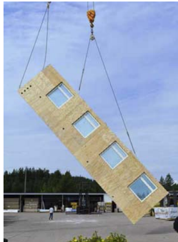
Figure 1-43 The horizontally manufactured element is turned into vertical position for assembly.
