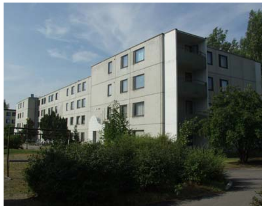
Figure 1-42 The situation prior to refurbishment. A four storey building with a facade made of concrete panels [Paroc Group Oy].
