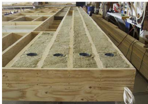
Figure 1-46 The manufacturing of the element in the workshop. The top connections of the ductwork, that will be connected to the AHU, can be seen [Paroc Group Oy].
