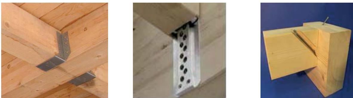
Figure 1. Typical joist connections for timber structures. From the left: joist hanger, dovetail connector, full thread screw.
