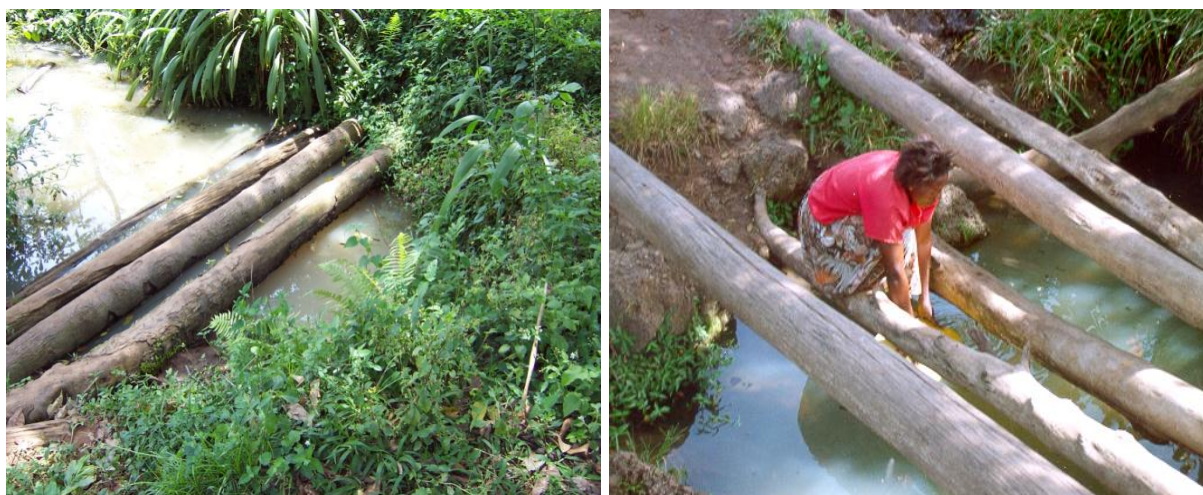
Photo 7: Example of Unprotected Shallow Wells Providing Water to Local Community
