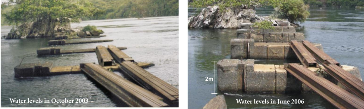
Photo 8: Sharp Decline in Water Levels in Lake Victoria
