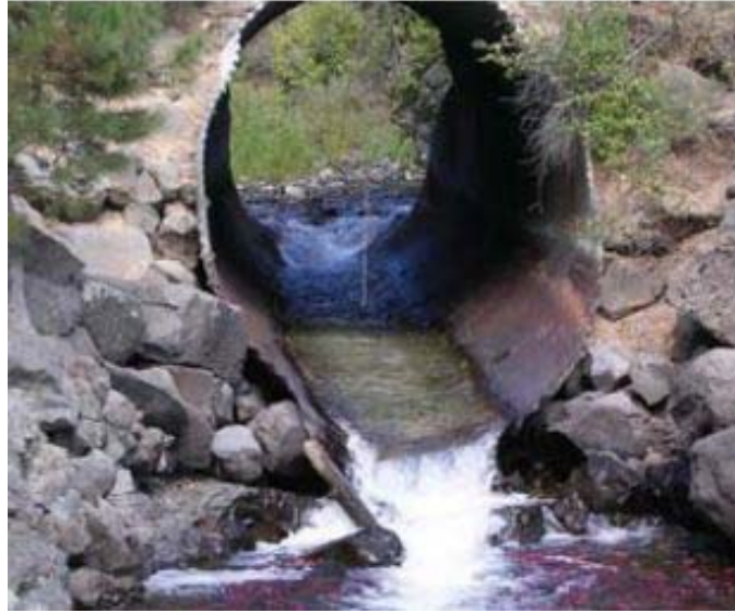
Figure 2.2: Culvert fishway (Forest Service Stream-Simulation Working Group, 2008).
