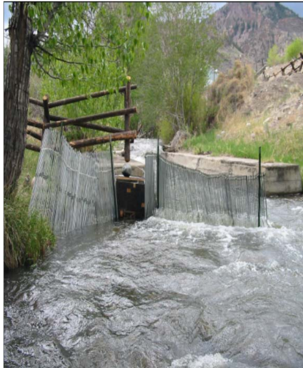
Figure A2: Fences that direct fish to the opening of trap #1 (after Blank, 2008).
