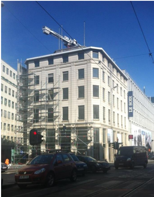
Figure 9: The building during the renovation in April 2013
