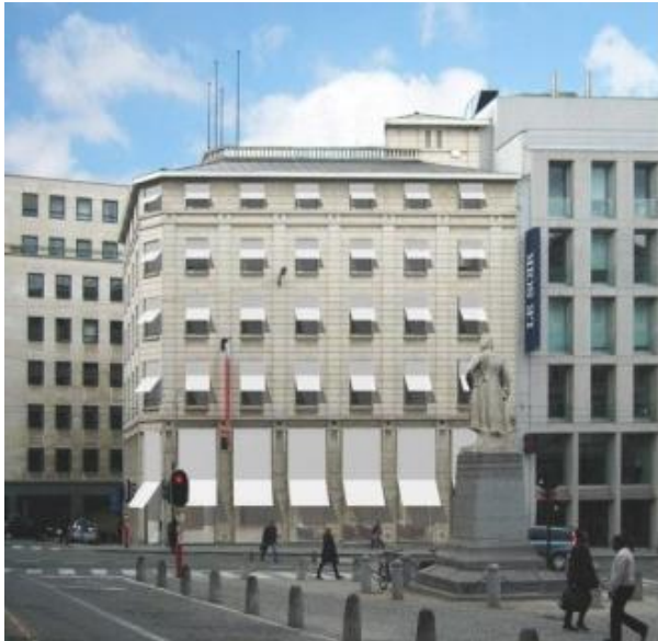
Figure 4: The façade with the external solar blinds.
