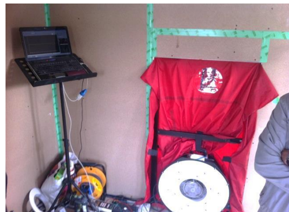
Figure 6: Blower test door during the site installation.
