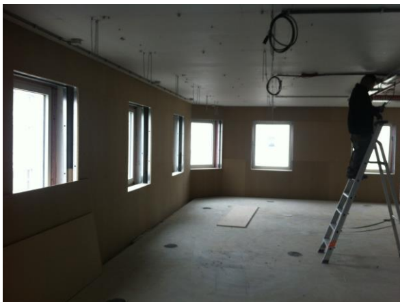
Figure 10: The building with the inner insulation in progress
