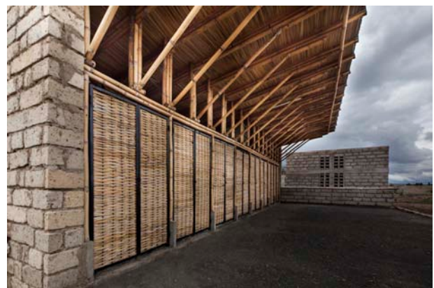
Figure 4: Façade of the workshop building: a hard shell of natural stone wall protects the soft core made of bamboo.
