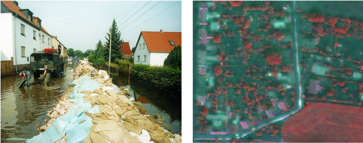
Figure 57. A temporary dam built on the road (left: in-situ photo, right: IKONOS imagery)
